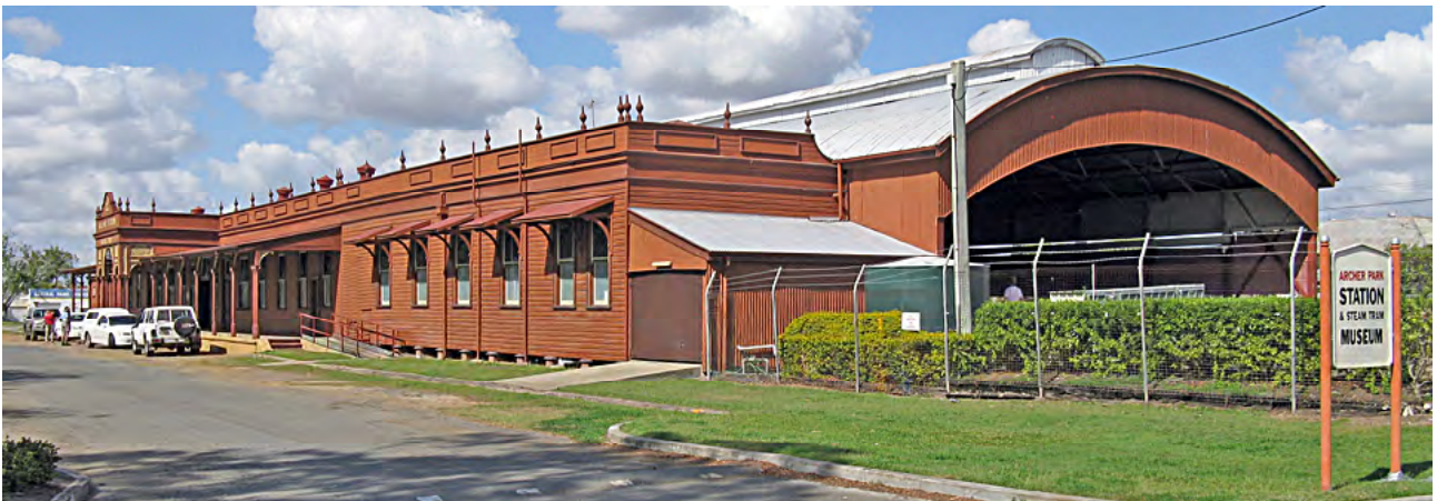
Cambridge Street entry to the station precinct. The refreshment rooms are on this end of the station and used to have a 'hole in the wall' service point for locals. The typical QR station carriage shade roof behind covers the platform and first two tracks, August 2009. [lz 4487]
