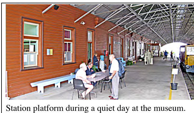
Station platform during a quiet day at the museum. The station was added to Queensland's Heritage Register 21 October 1992, underwent four years of restoration begun in 1996, and opened as a volunteer operated museum 11 December 1999.
