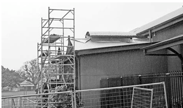
Men's toilet area of the roof while under repair early June.
