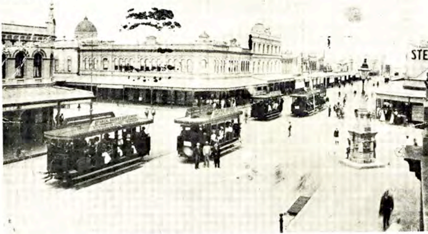
East Street, Rockhampton around 1912. Cars 7 and 8 are closest to the camera, the air hose connections for the trailer's brakes can be seen. The trams are carrying roof destination boards and auxiliary signs on the aprons.
